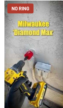
Drill through a Stucco Wall for LB fitting and wire pulling
